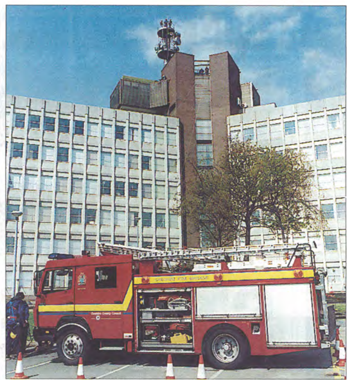
Head Office tower – the task facing the rescuers.
